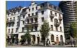
GAIA HOTEL Switzerland
